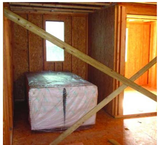
**Figure 5** Pack of plasterboards placed within a structure as erection proceeds
