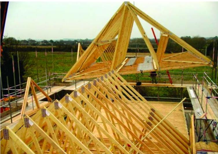
**Figure 7** Lifting pre-assembled trussed rafter roof sections
