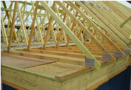
**Figure 6** Temporary fixing of trussed rafters on the safe working platform of a lower deck
