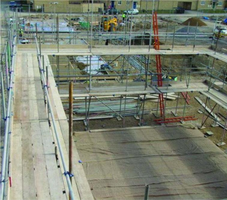
**Figure 4** Scaffolding in place before erection of the frame
