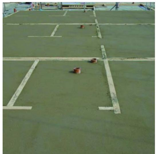
**Figure 3** Screeded base with sole plates in position
